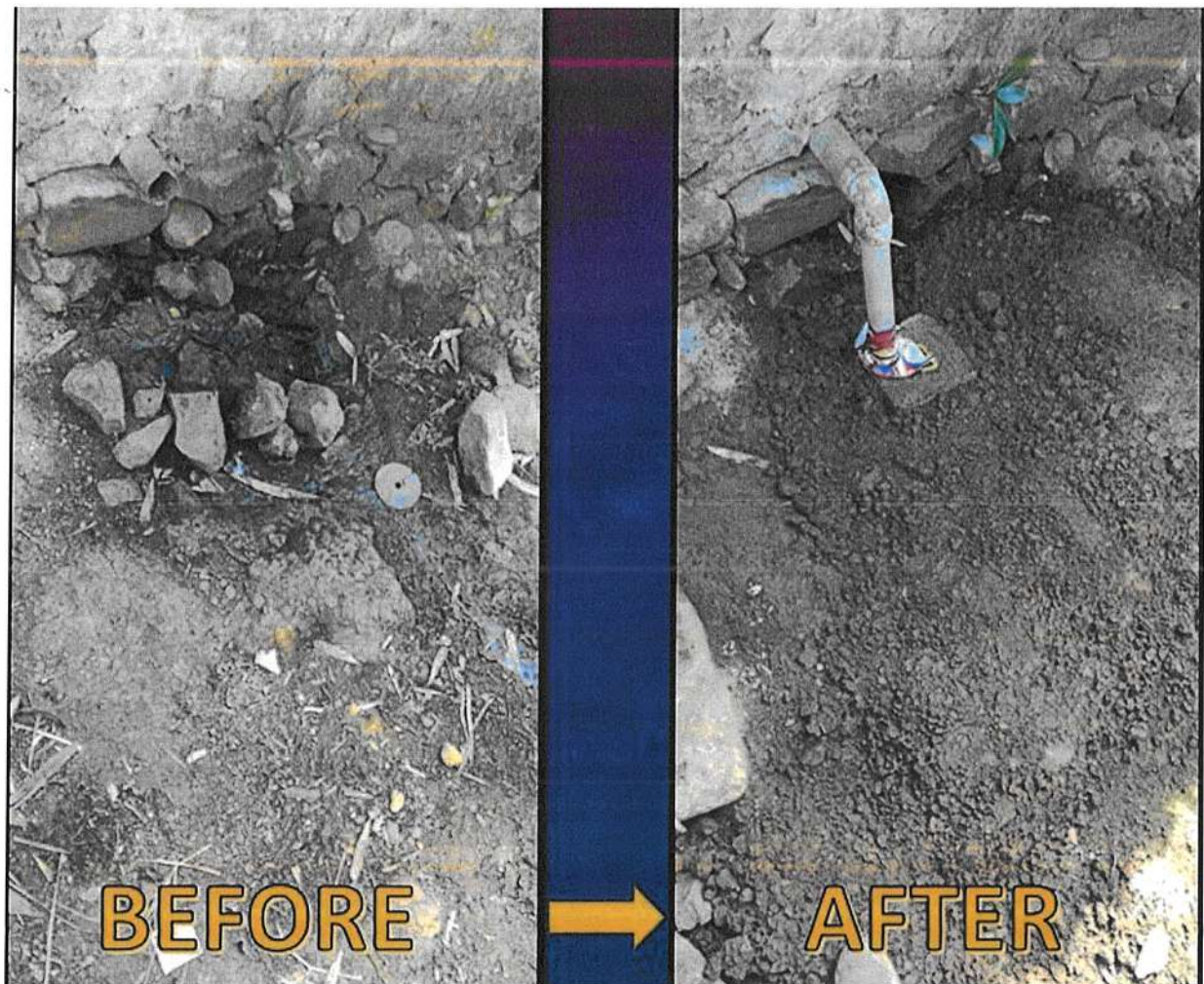
Soak-pit Construction Work
